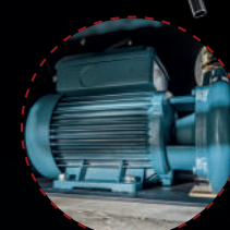
PUMP: External discharge pump
